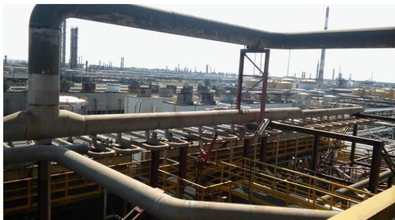
**Picture 2 (top):** view of stream 1 line coming from the top and splitted in 2 700 mm lines
