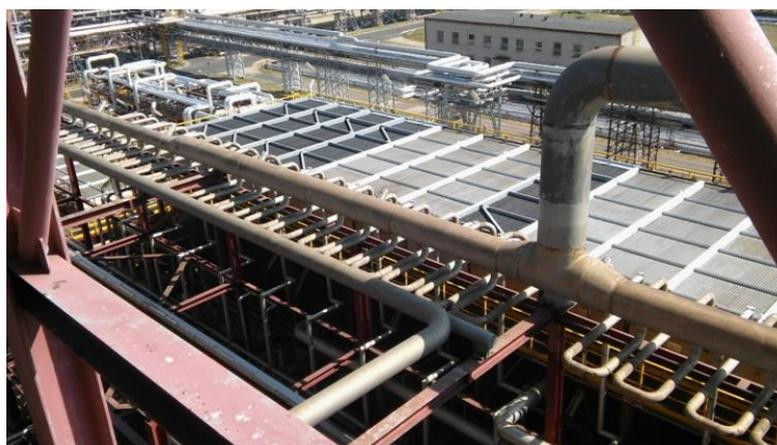
**Picture 3 (bottom):** alternate view of the split of stream 1 and the air cooling units
