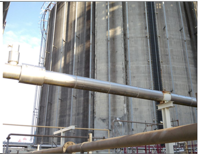
Picture 1 of the pipe section
